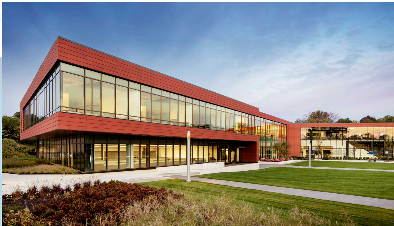
Our Lowell, Massachusetts facility (pictured above) includes our primary operations and manufacturing capabilities, as well as our corporate headquarters, and represents more than 30% of our worldwide headcount and global footprint. (See page 21 for our worldwide locations.)
